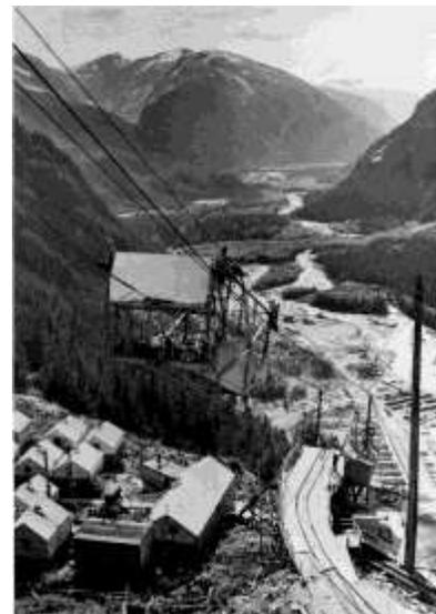
*Figure 4: The tramway that carried material, supplies and crews up to the work stations.*
