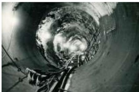
*Figure 3 : 21-foot diameter hole in the mountain with the penstock in construction.*
