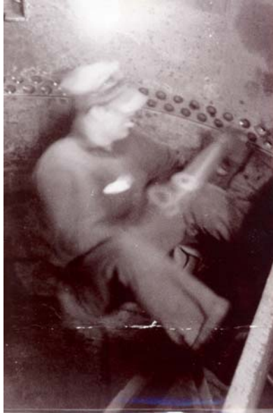
Figure 5 - In the early 1940's the skill of riveting was still in demand. Riveting required five men to close up a seam compare to one welder.
