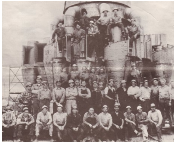
Figure 6 – Cat cracker in Sarnia, Ontario for Imperial Oil, 1956
