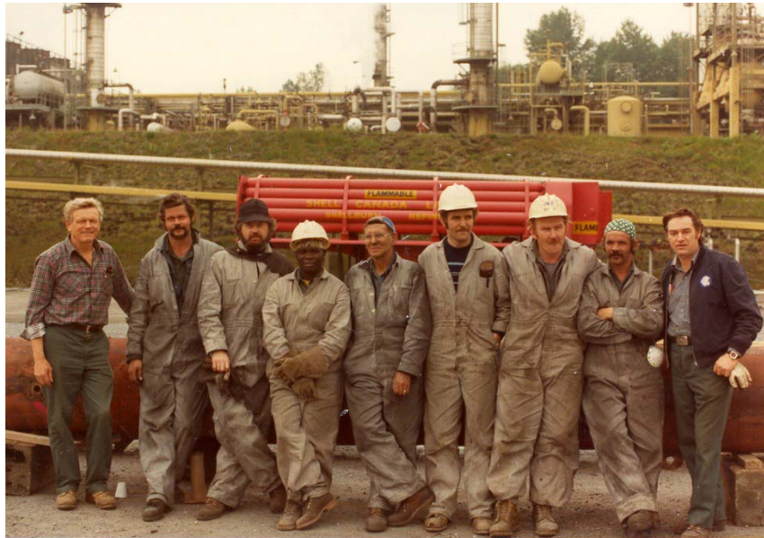
Figure 8 –Constructing, maintaining and repairing the Industrial landscape of Canada is the work of the Construction Boilermaker.
