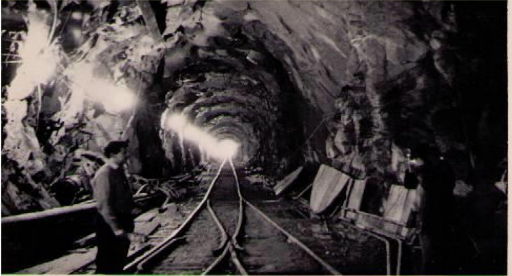
The penstock cans were fabricated in Vancouver then shipped out to Kemano and installed in the tunnels on an incline of 48 degrees making for very dangerous and uncomfortable working conditions.
