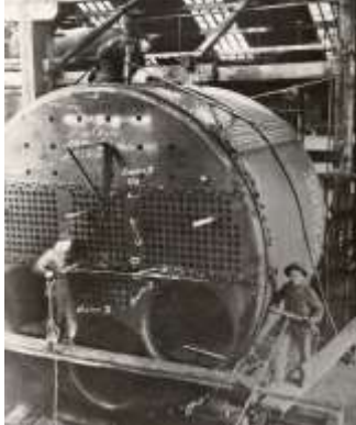
Figure 2 Mechanics using air guns, very loud work with a lot of vibration. Caused Boilermaking hearing and white knuckle disease.
