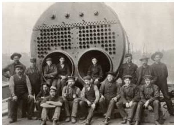
Figure 1 - Proud Boilermakers with a finish product. Note the young people, photo taken at the same time Percy Wilson started his apprenticeship in 1900.
